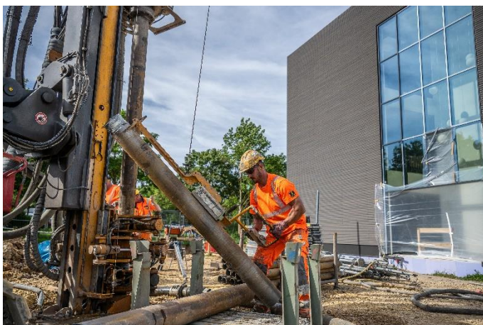
(2) 24 geothermal probes were installed in a very confined space.
