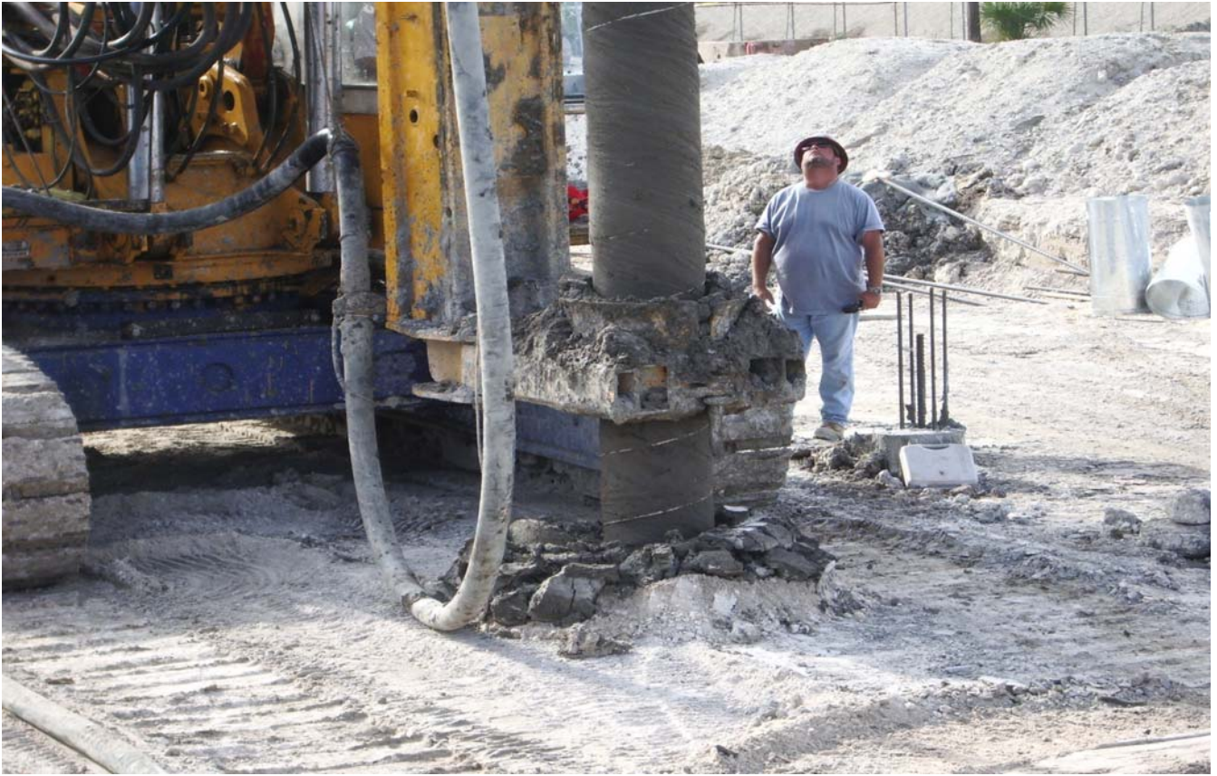
Grout Installation through Continuous Flight Auger
