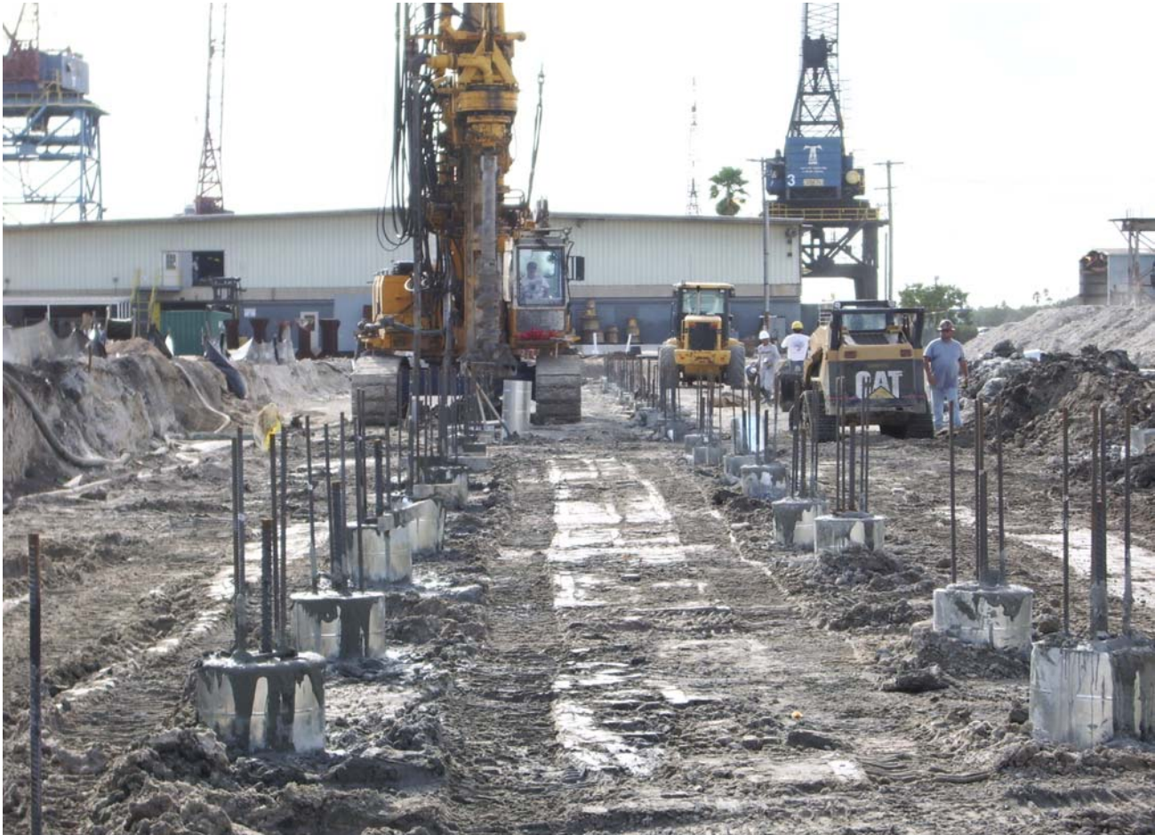
BG 22 Drill Rig
