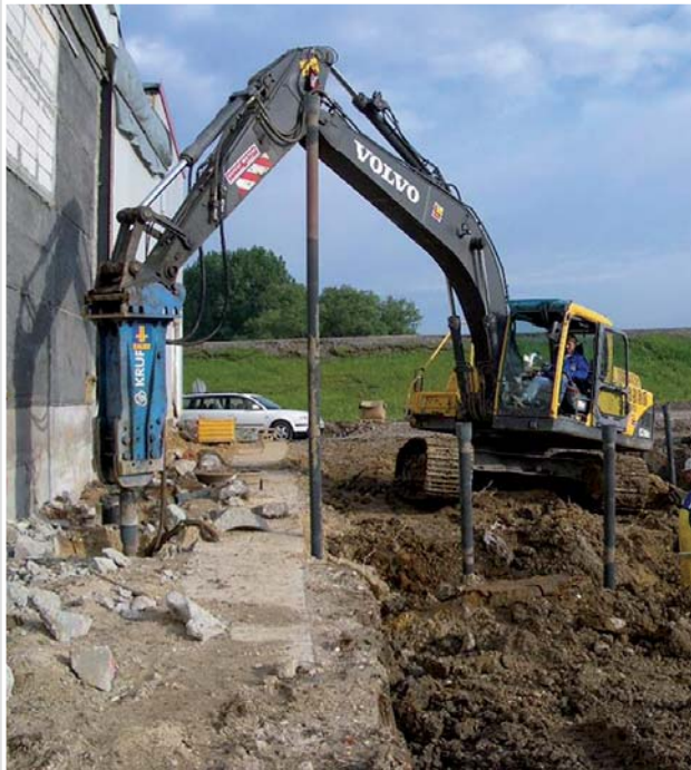
Foundation works adjacent to an existing building
