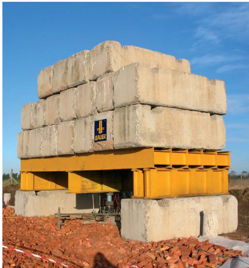
Static pile test
