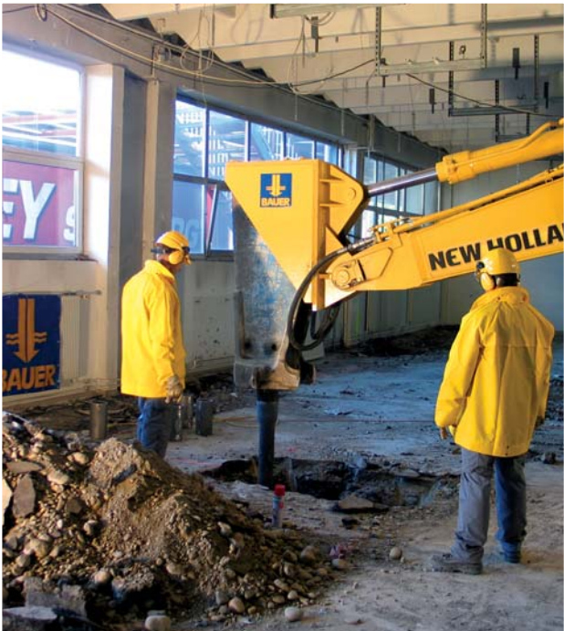
Underpinning works in restricted headroom
