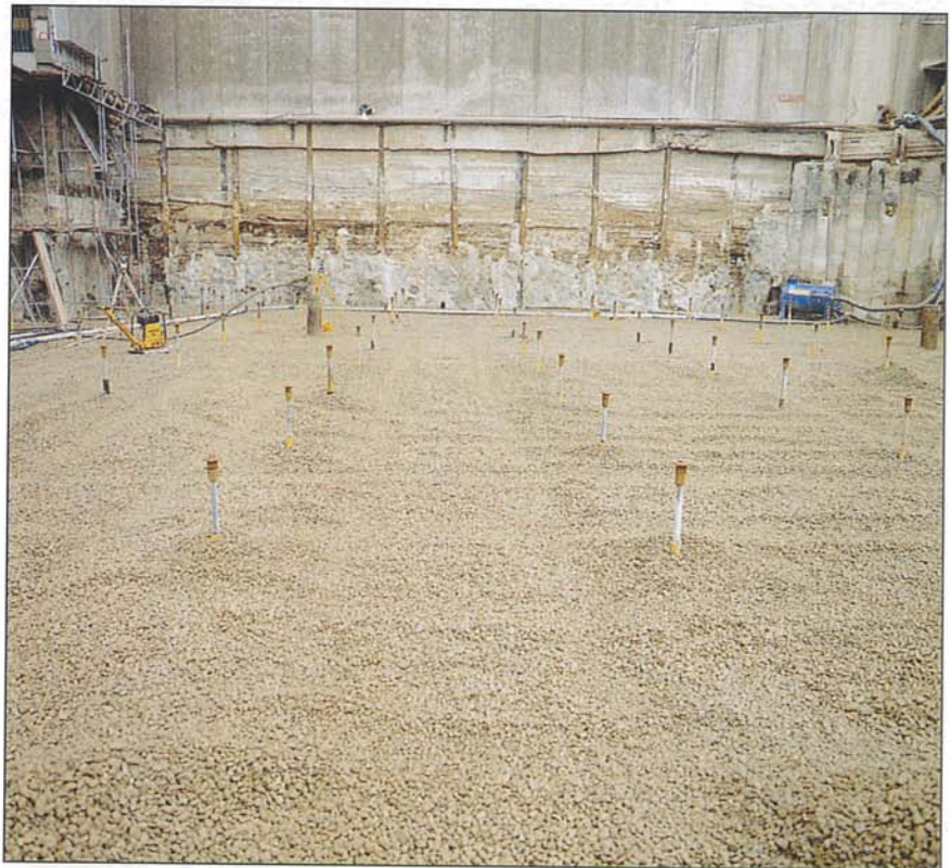
Anchored jet grouted base slab
