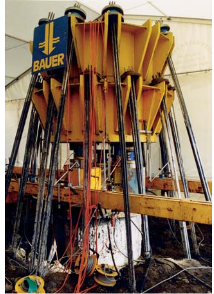
Pile test below tent at Daun upon Eifel
