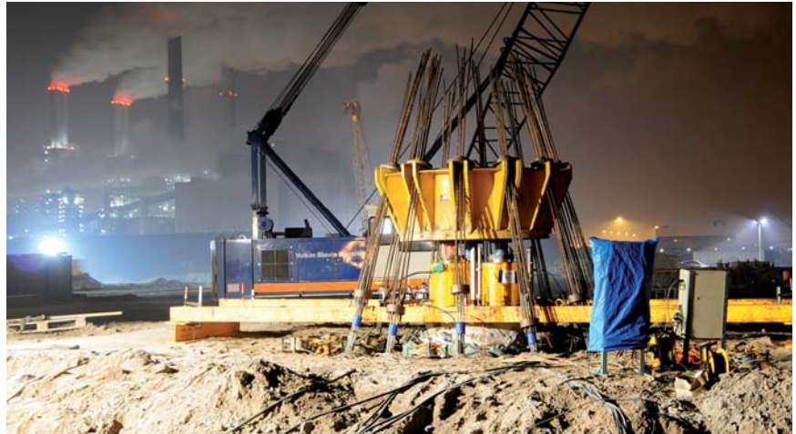
Pile test in Rotterdam-Maasvlakte, Netherlands for E.ON power station
