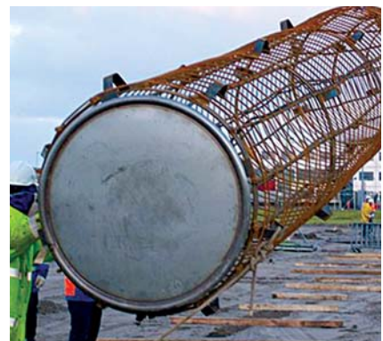
Bauer Lift-Cell to pre-stress the pile bottom
