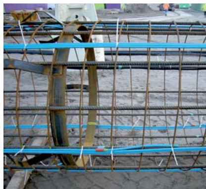
Injection hoses for skin grouting
